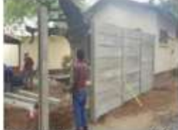
Precast Compound Wall
