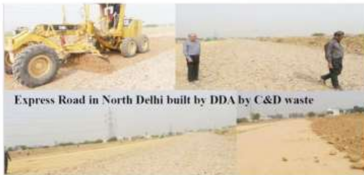
Road constructed with C&D waste processed material at Delhi
