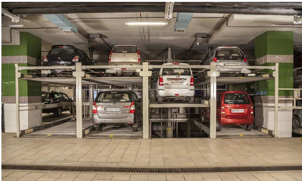
Figure 6.8: Multi-level car parking (example)
