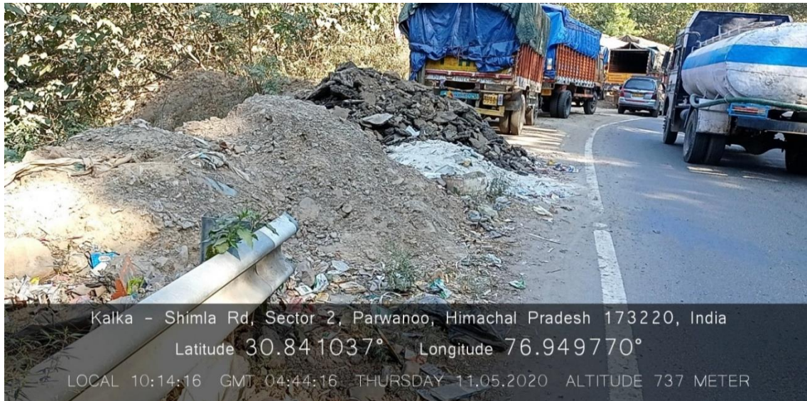
Figure 4.25: Construction and Demolition debris near construction sites
