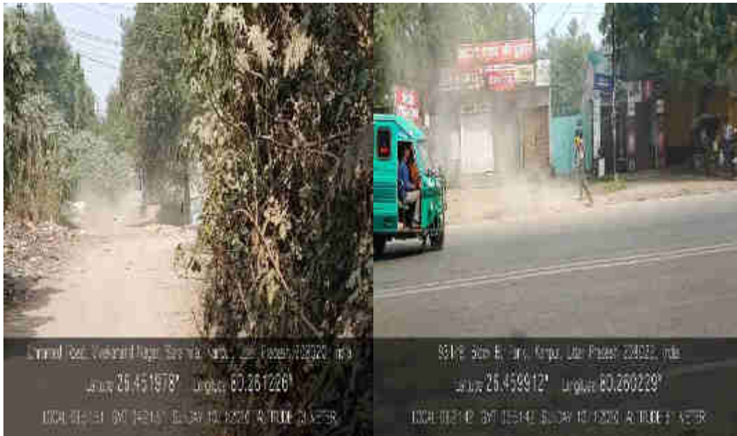
Figure 3.99: Road dust deposition on the paved road
