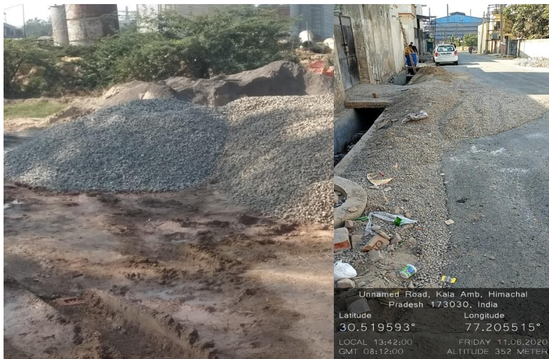
Figure 4.24: Construction material and debris near construction sites
