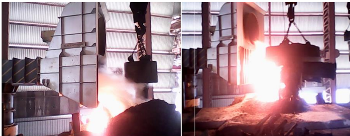
Figure 6.13: Working on side-based Suction Hood (Sharma, 2020)
