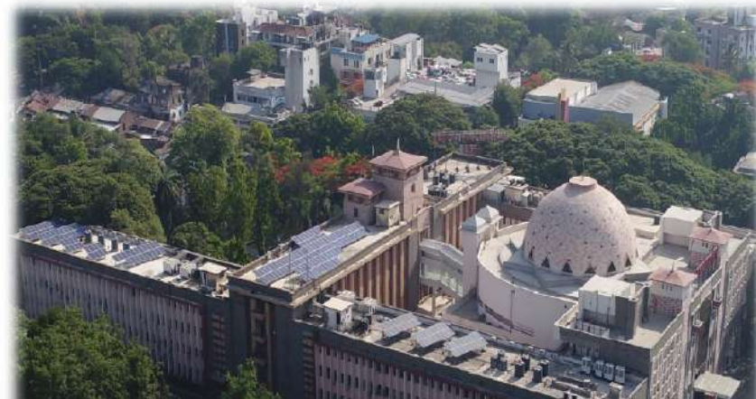
Installation of Solar Panels on PMC Building
