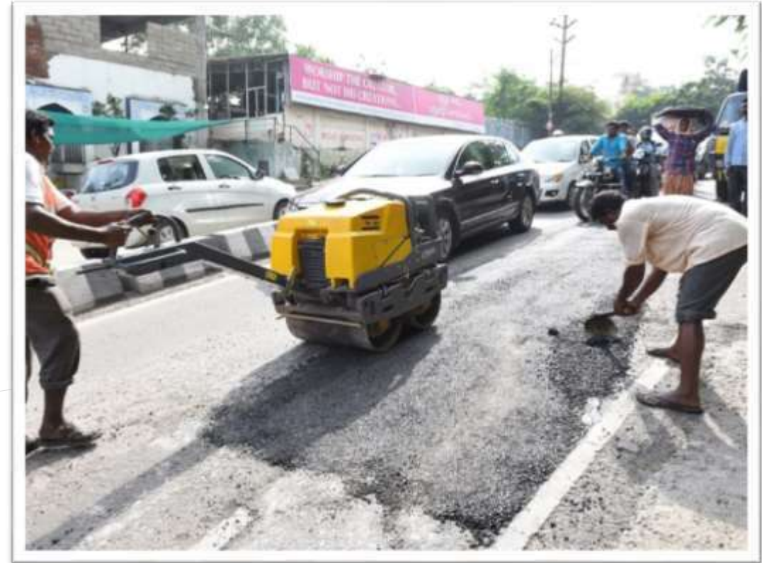
Pothole Maintenance
