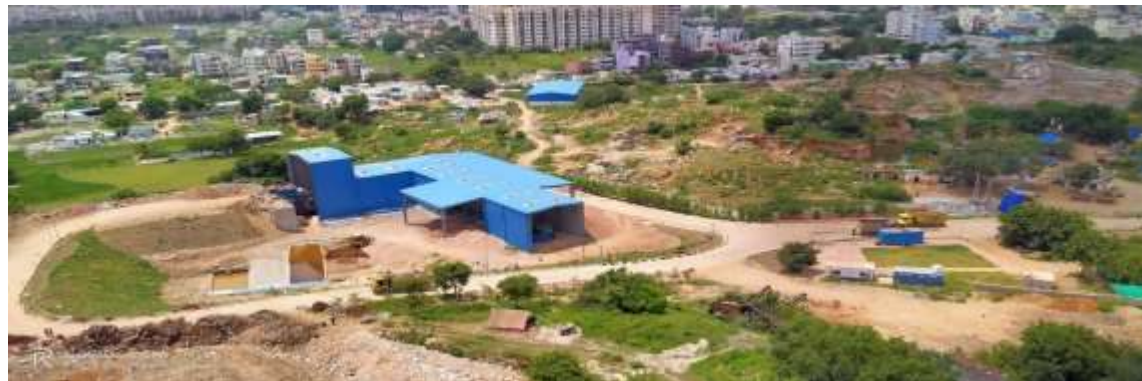
C&D waste recycling plant at Jeedimetla
