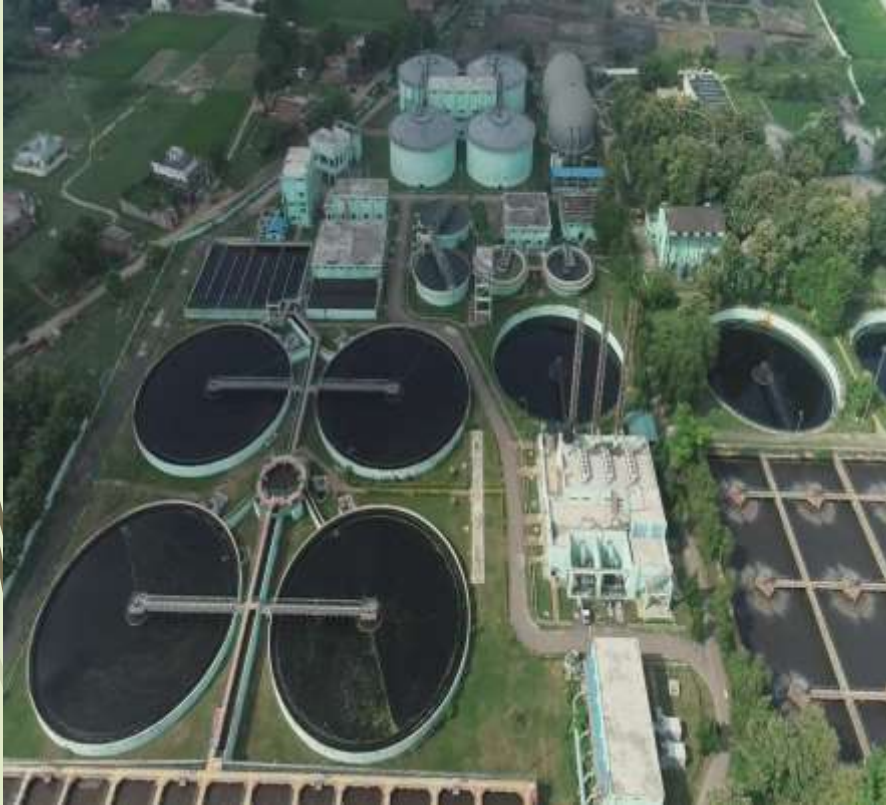
140 MLD STP Plant at Dinapur
