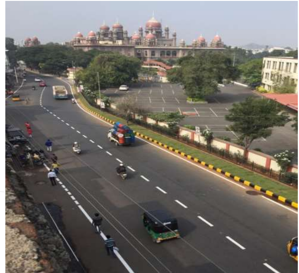
CRMP Road besides High Court of Telangana
