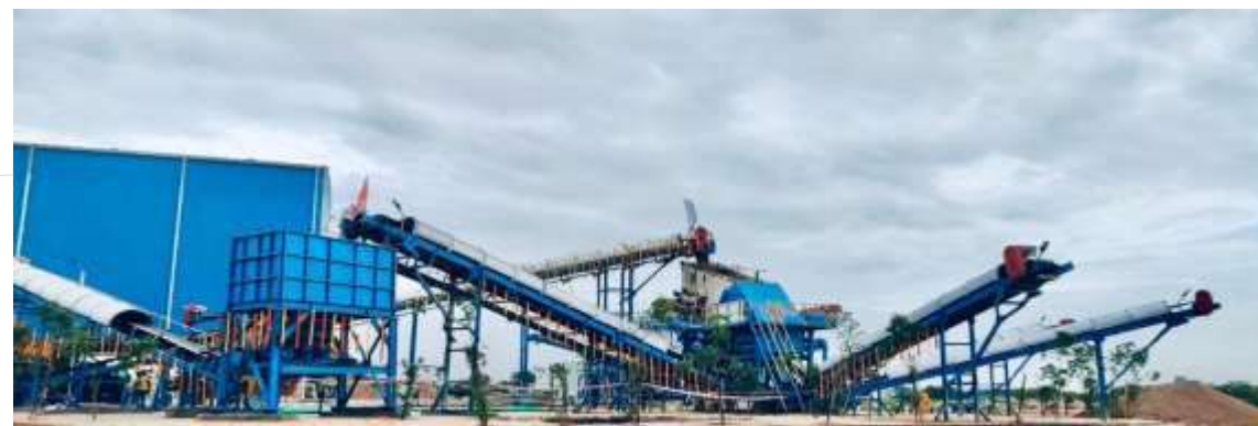
C&D waste recycling plant at Fatullaguda
