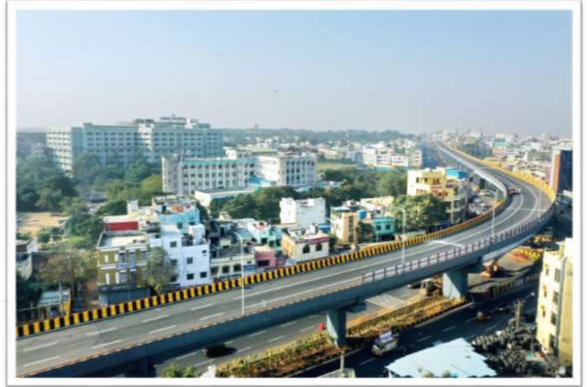
Flyover at Owaisi Hospital Junction
