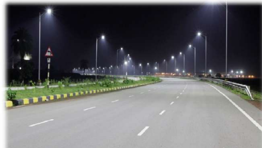
Installation of 1,80,000 LED Street Lights
