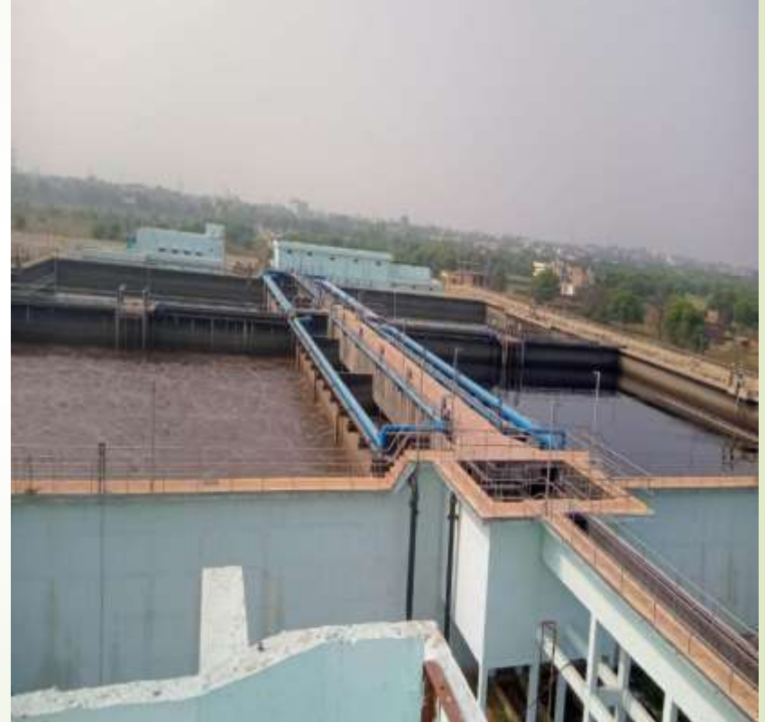
50 MLD WTP Plant at Ramna
